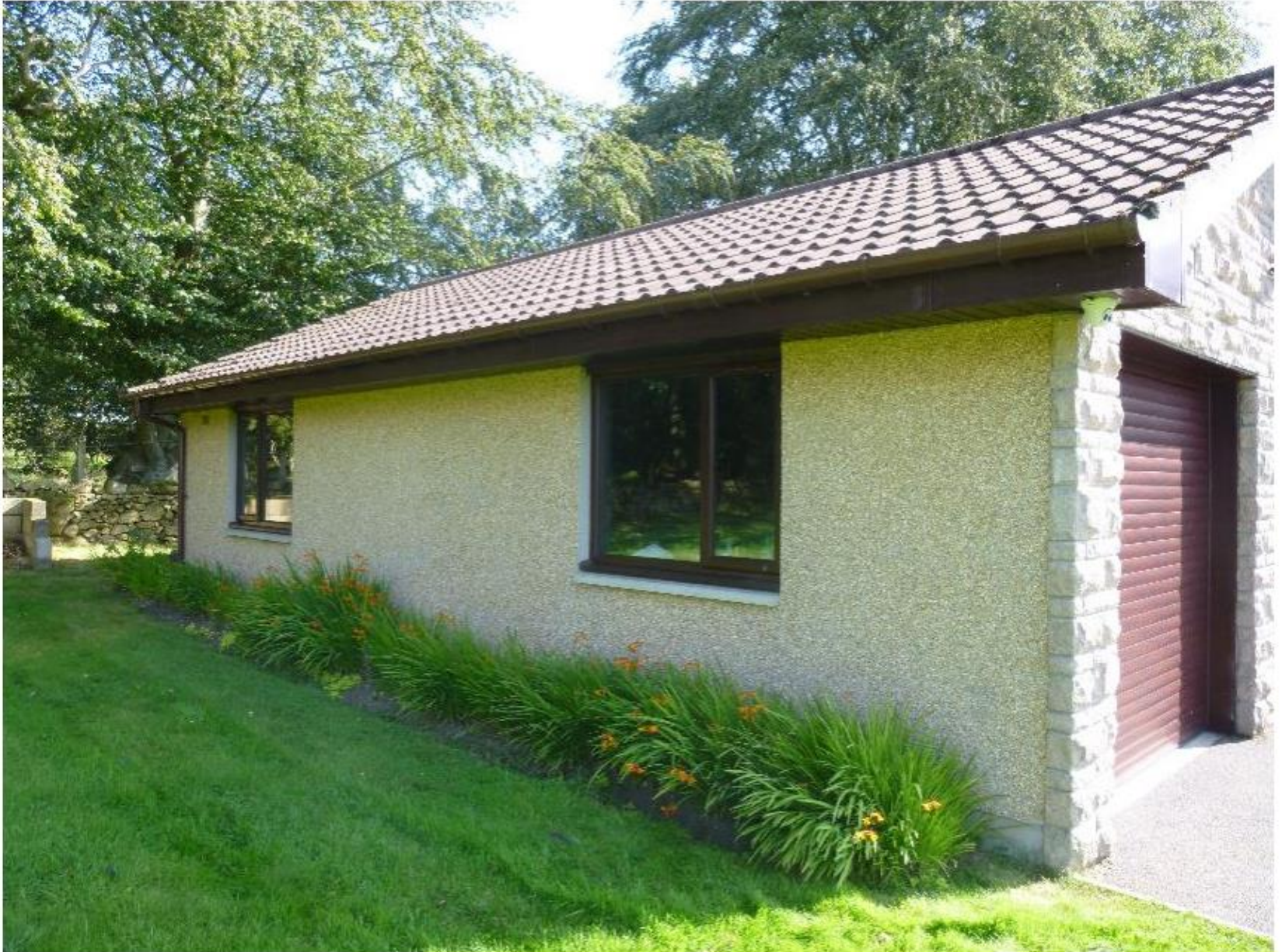
Photo: Existing Garage (side)
